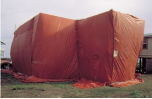
Figure 10. Covered structure fumigation.
